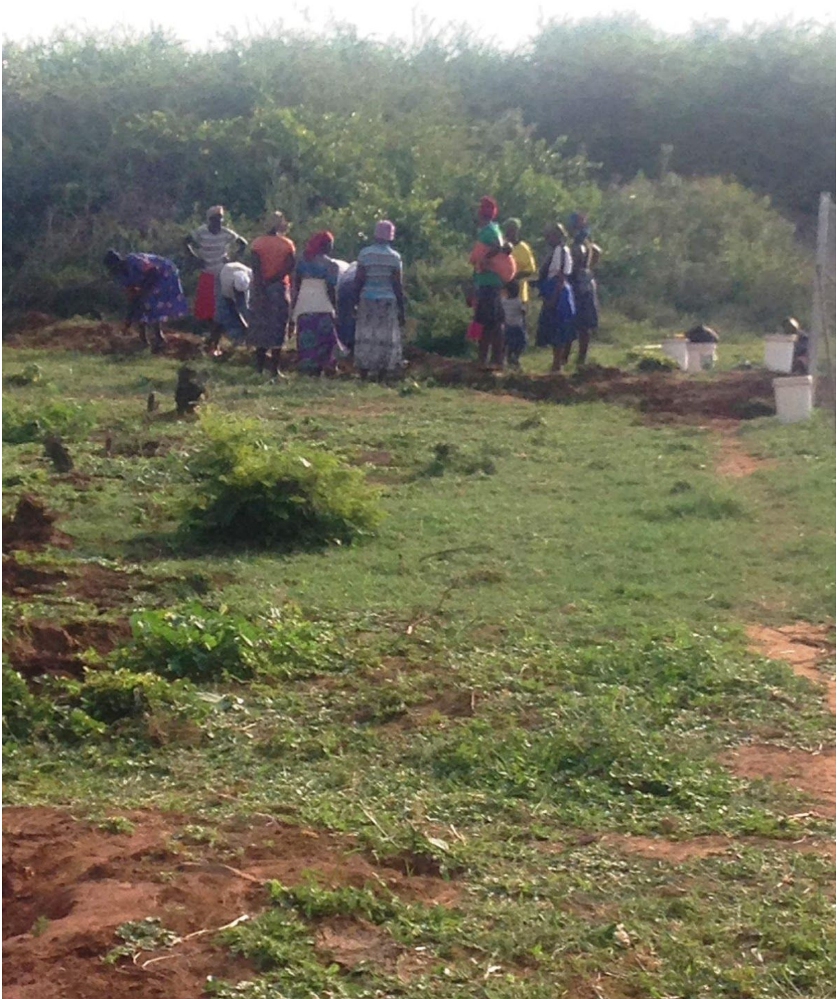
Women burying the pipes after system completion
