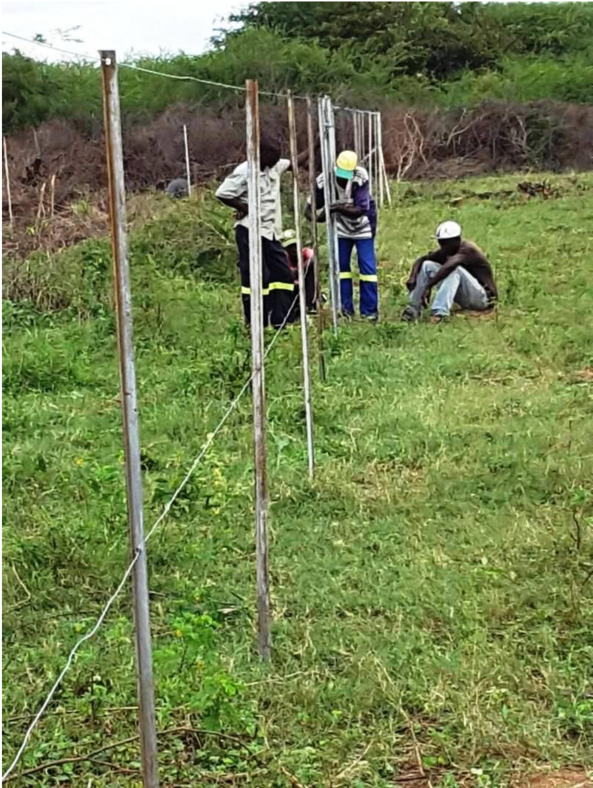
Fencing was commenced at Tamuka Garden on 10 April 2018
