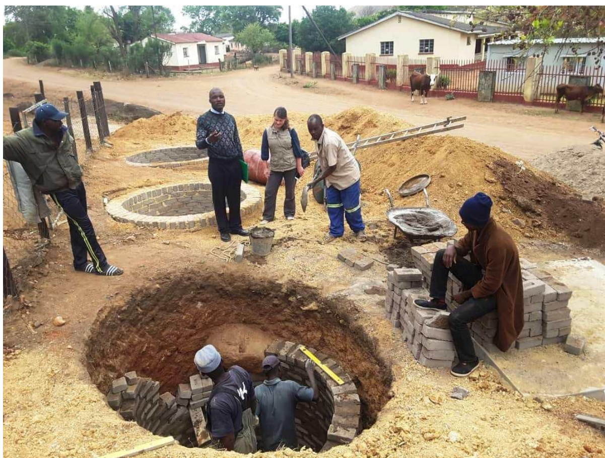
State of the incinerator project as at October 27 th
